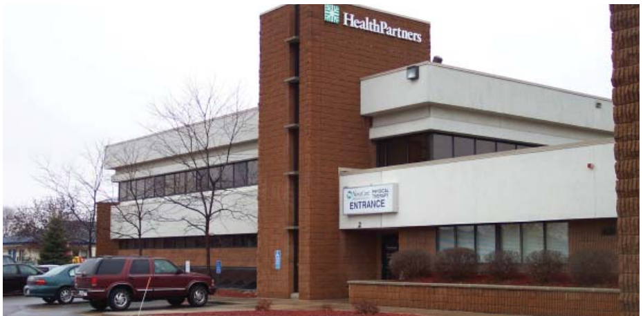
South elevation of building to be renovated for Allied Health.
