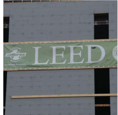
LEED certification is being pursued at Wellness Center.
